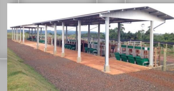
Feedlot facilities of the Center for Tropical Research in Water Buffalo (CPTB), Botucatu, São Paulo, Brazil.
