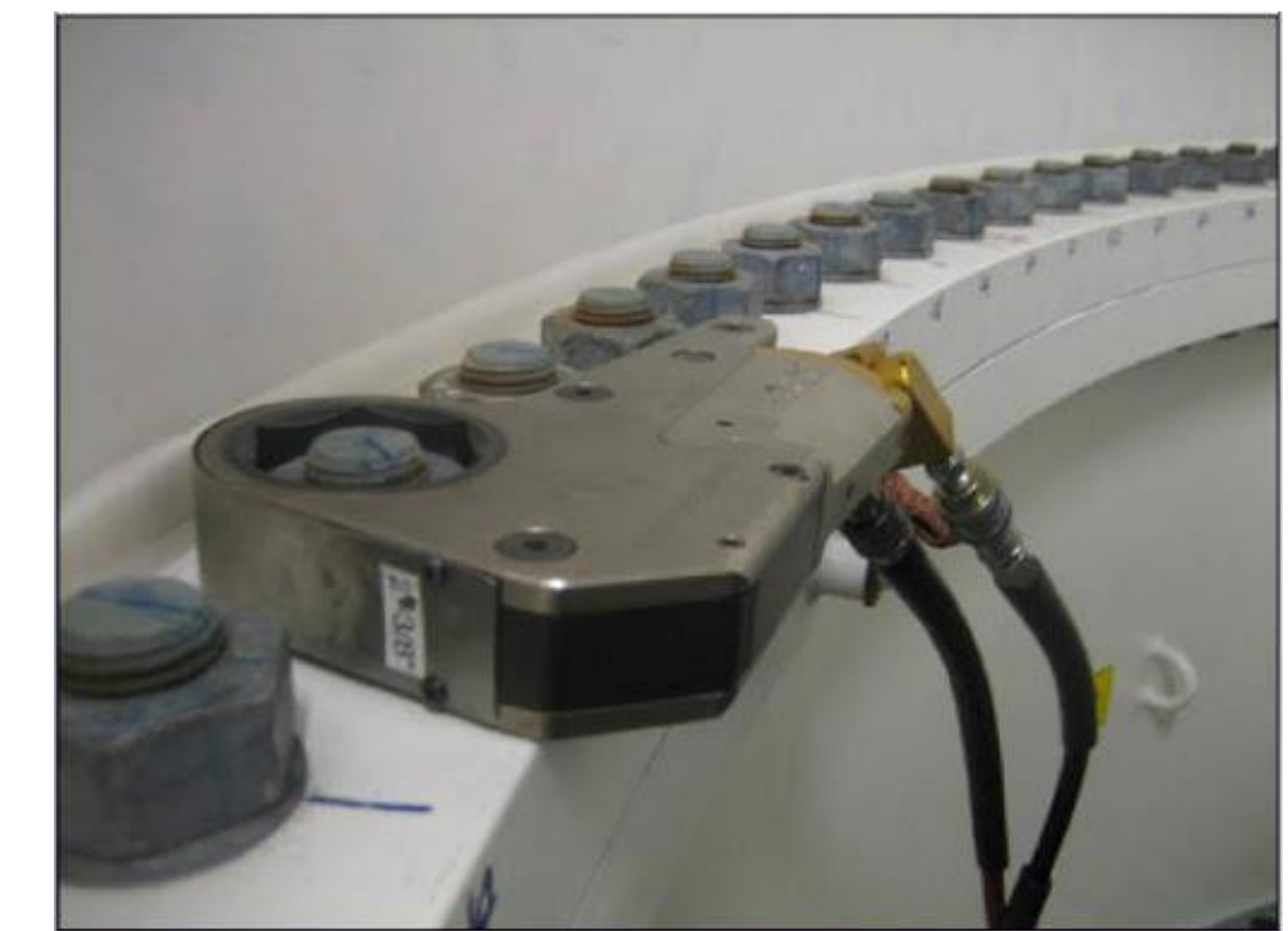
Right: Torque wrench on wind turbine flange bolts
